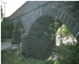
1 bridge over merri creek coburg side view
