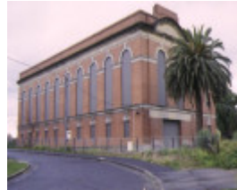
1 railway sub station off newmarket street flemington front view
