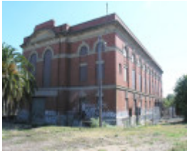
RAILWAY SUB-STATION SOHE 2008
