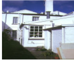
162 cyprus terrace external rear view
