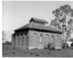
H1053 1 echuca pumping station 1964 slv
