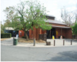
FORMER PUMPING STATION SOHE 2008
