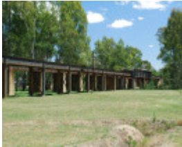
RAIL BRIDGE SOHE 2008
