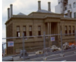
1 customs house geelong ac may00
