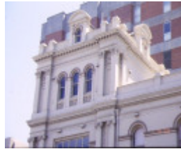
aubrey bowen wing royal victorian eye & ear hospital morrison place east melbourne facade detail jan1998
