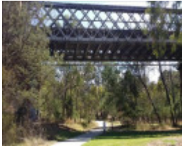
Chandler Highway Bridge
