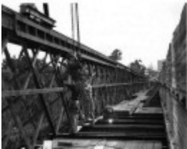
Chandler Highway Bridge construction works .jpg
