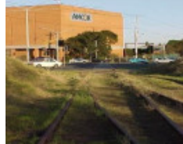
Tracks at the former site of the Fulham Grange Station (now removed) approaching the Chandler Highway Bridge.jpg
