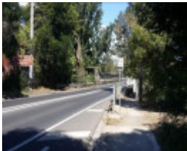
Chandler Highway Bridge looking to the south (City of Boroondara) from the northern side of the bridge (City of Yarra).jpg
