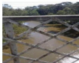
A detail of the cantilevered walkway looking west along the Yarra River.jpg
