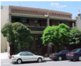
1 terrace 22 morrison place east melbourne front view oct1999
