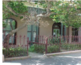
terrace 22 morrison place east melbourne front elevation oct1999
