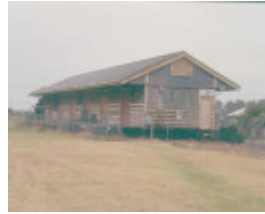
h02072 port fairy goods shed
