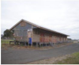
RAILWAY GOODS SHED SOHE 2008
