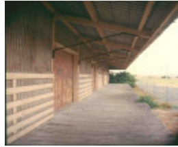
h02072 port fairy goods shed platform
