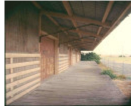
h02072 port fairy goods shed platform
