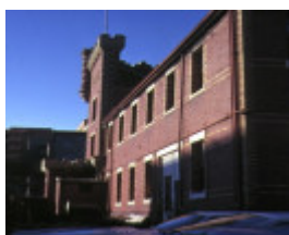
former salvation army training garrison victoria prd east melb front wall jul1982
