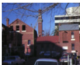
former salvation army training garrison victoria prd east melb rear view jul1982
