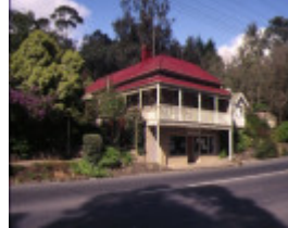
1 former warrandyte wine hall yarra street warrandyte front view
