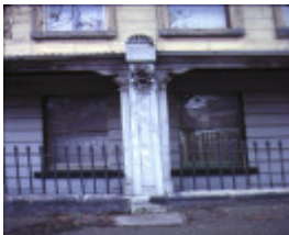
terrace 352 354 victoria parade east melbourne pillar detail jul1980
