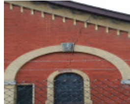
FORMER RAILWAY ENGINE SHED SOHE 2008
