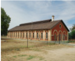
FORMER RAILWAY ENGINE SHED SOHE 2008
