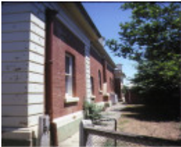
echuca court house side elevation dec1983
