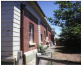
echuca court house side elevation dec1983
