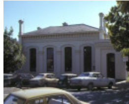
former echuca town hall rear view may1979
