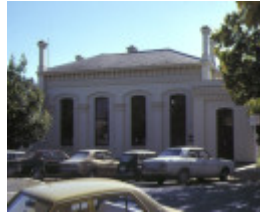
former echuca town hall rear view may1979
