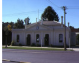
1 former echuca town hall front view may1979
