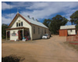
506-508 Napier Street, White Hills Uniting Church & Hall
