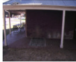
hopwood hotel echuca verandah
