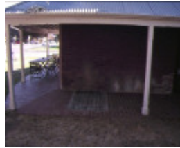
hopwood hotel echuca verandah
