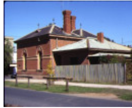
former customs house echuca side view
