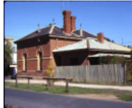
former customs house echuca side view
