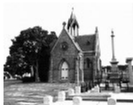
038 - Cemetery Chapel, Carpenter St_Page_1.jpg
