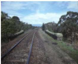
rail bridge & embankment geelong ballarat line elaine rail detail
