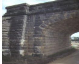
rail bridge & embankment geelong ballarat line elaine arch detail aug 84
