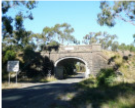
RAIL BRIDGE AND EMBANKMENT SOHE 2008
