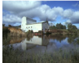
eldorado bucket dredge byawatha road eldorado site view
