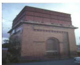
elmore railway station & water tower water tower front view
