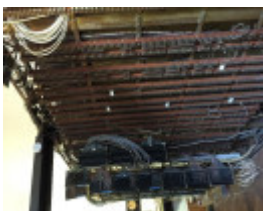
EASTERN HILL FIRE STATION July 2016
