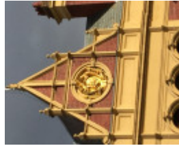
EASTERN HILL FIRE STATION July 2016
