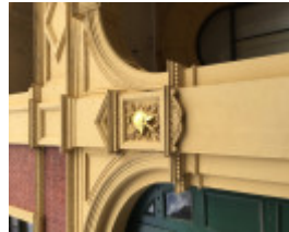
EASTERN HILL FIRE STATION July 2016
