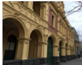
EASTERN HILL FIRE STATION July 2016
