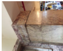
EASTERN HILL FIRE STATION July 2016
