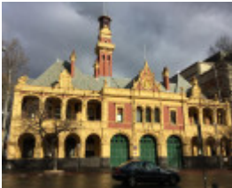
EASTERN HILL FIRE STATION July 2016
