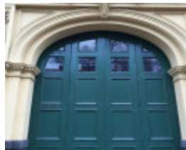
EASTERN HILL FIRE STATION July 2016
