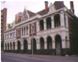
1 eastern hill fire station victoria parade east melbourne front view feb1994
