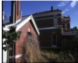
former elsternwick post office rear view
