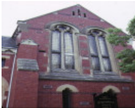
former union church elsternwick front window detail
