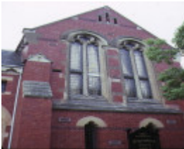
former union church elsternwick front window detail
