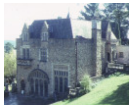
montsalvat hillcrest avenue eltham view of windows
