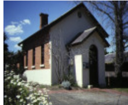
eltham court house main road eltham front corner elevation
