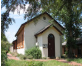
ELTHAM COURT HOUSE SOHE 2008
