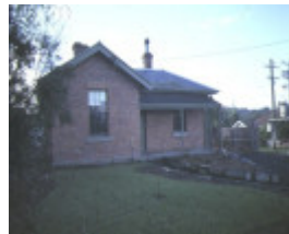
1 former police quarters main road eltham front view apr1986
