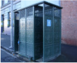
Urinal Queensberry & Elizabeth St exterior KJ 21 06 2007
