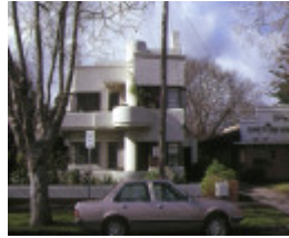
1 windermere flats broadway elwood front elevation jul1989
