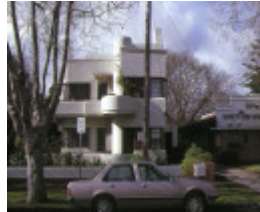
1 windermere flats broadway elwood front elevation jul1989
