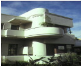
windermere flats broadway elwood detail of central curves
