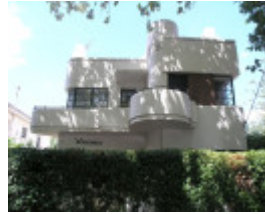
WINDERMERE FLATS SOHE 2008
