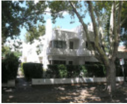
WINDERMERE FLATS SOHE 2008
