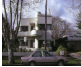
1 windermere flats broadway elwood front elevation jul1989
