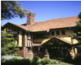
1 hartpury court complex milton street elwood front view nov1998
