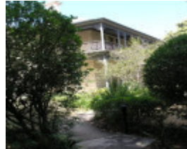
HARTPURY COURT COMPLEX SOHE 2008
