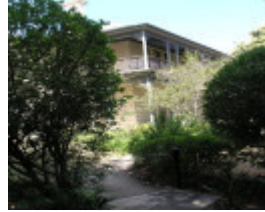
HARTPURY COURT COMPLEX SOHE 2008
