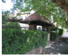
HARTPURY COURT COMPLEX SOHE 2008
