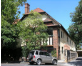
HARTPURY COURT COMPLEX SOHE 2008
