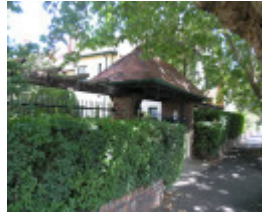
HARTPURY COURT COMPLEX SOHE 2008
