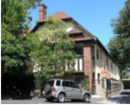
HARTPURY COURT COMPLEX SOHE 2008
