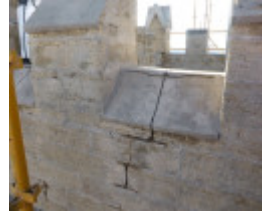
Before Photograph - Reference F3866 2014
