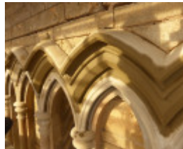
During Photograph - Reference F3866 2015
