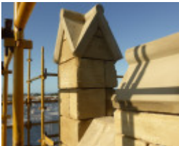
During Photograph - Reference F3866 2015
