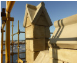
During Photograph - Reference F3866 2015
