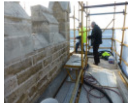
During Photograph - Reference F3866 2015
