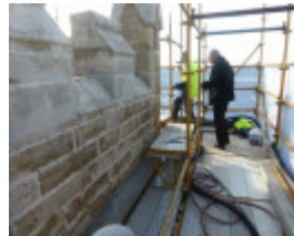
During Photograph - Reference F3866 2015
