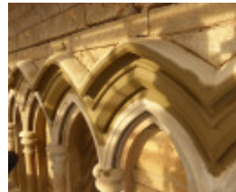
During Photograph - Reference F3866 2015
