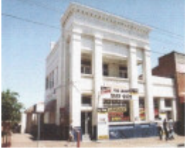
State Savings Bank 438 Centre Rd Bentleigh
