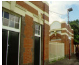
essendon railway station complex store buildings sw oct 1998
