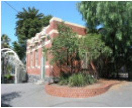
ESSENDON RAILWAY STATION COMPLEX SOHE 2008
