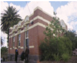
essendon railway station complex buckley street essendon street elevation oct1998
