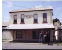
1 bacchus marsh express office & printing works front view
