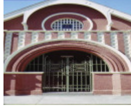
euroa courthouse detail of entrance
