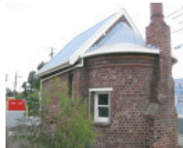
Former Ferry Terra Cotta & enamel brickworks office albert Street brunswick rounded end from the southeast
