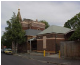
flemington post office wellington street flemington rear she project 2004
