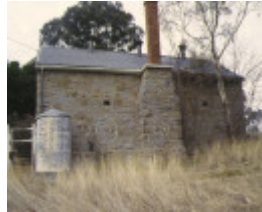
faraday primary school no 797 calder highway faraday rear view apr 97
