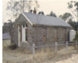
1 faraday primary school no 797 calder highway faraday corner view apr 97
