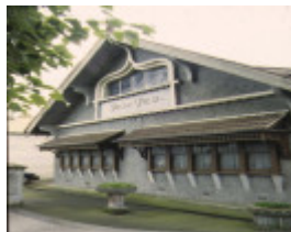
1 park view racecourse road flemington front elevation apr1996
