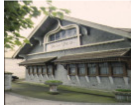
1 park view racecourse road flemington front elevation apr1996
