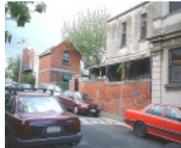
h01204 h1204 166 bellair st kensington general view of rear from south.jpg
