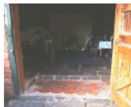
h01204 h1204 166 bellair st kensington rear stables floor recent slate
