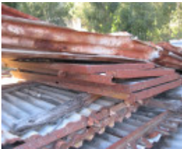
Porter prefabricated iron store
