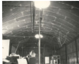
Porter prefabricated iron store
