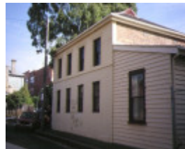
former national school bell street fitzroy building 2 1994
