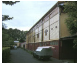
fitzroy cricket ground grandstand brunswick street fitzroy rear view may1993
