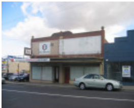
High Street Reservoir, No 763-765
