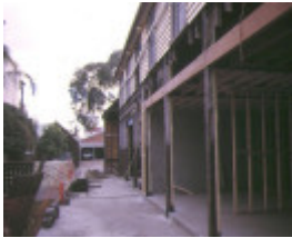
1 former richmond drill hall gipps street richmond rear view
