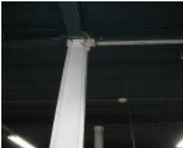
Dimmeys_Richmondinterior columns_9 July 08
