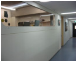
Plumbers & gasfitters ground floor corridor
