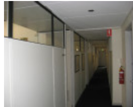
Plumbers & gasfitters second floor
