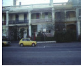
1 barcelona terrace brunswick street fitzroy front view 43 45 & 47 sep1978
