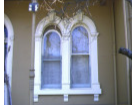
barcelona terrace brunswick steret fitzroy window detail
